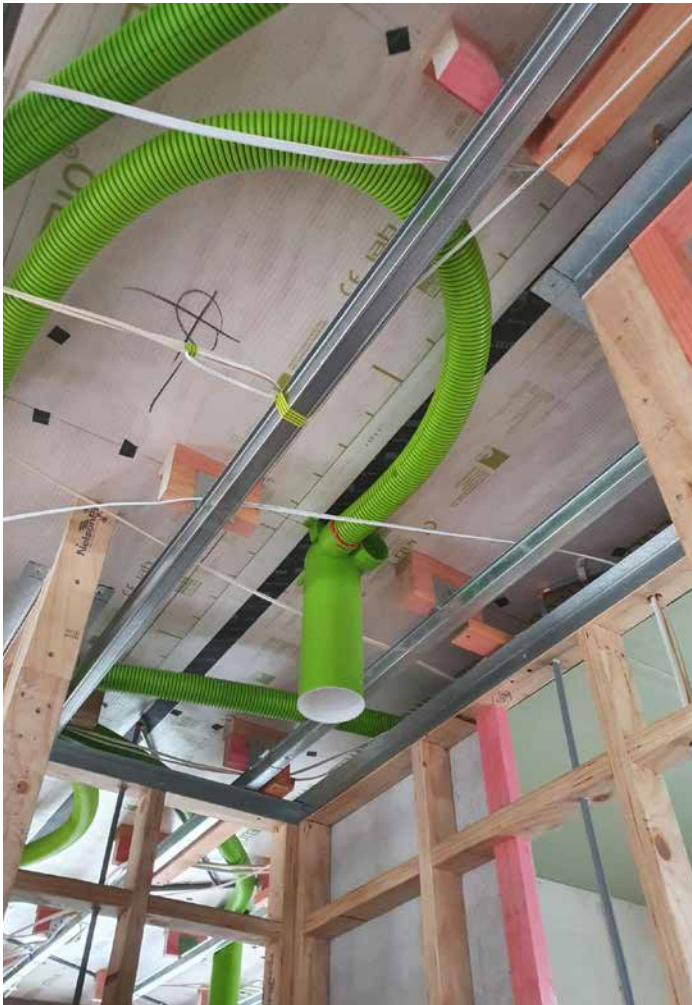
This ceiling service cavity neatly contains wiring, plumbing, MVHR ducting and the MVHR terminal (outlet to the room).
