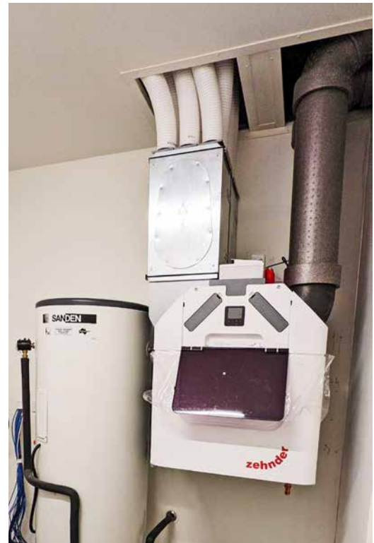
MVHR units aren't large. In a single-family home, they are often located in a cupboard in the laundry. In apartments, an MVHR unit might fit in a kitchen cupboard.
